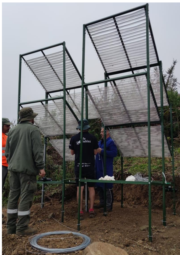
Fig. 56. Modular i-FWC being installed in El Pinillo (Valleseco, Gran Canaria).
